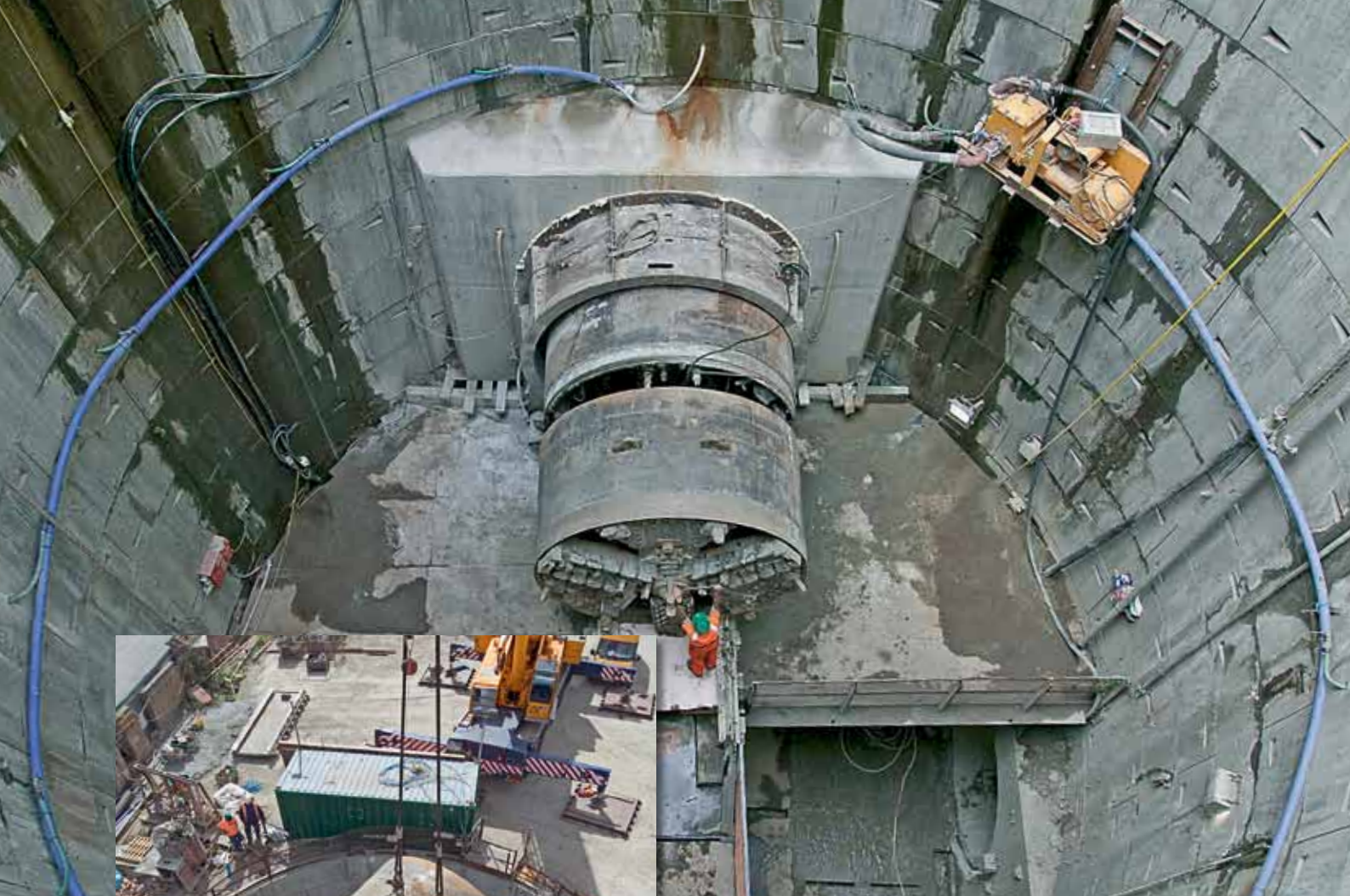
▲ "Helen," a 2.82 tunnel boring machine, with the EDF Energy tunnel below. Shows the de-watering tubes and pumps.
