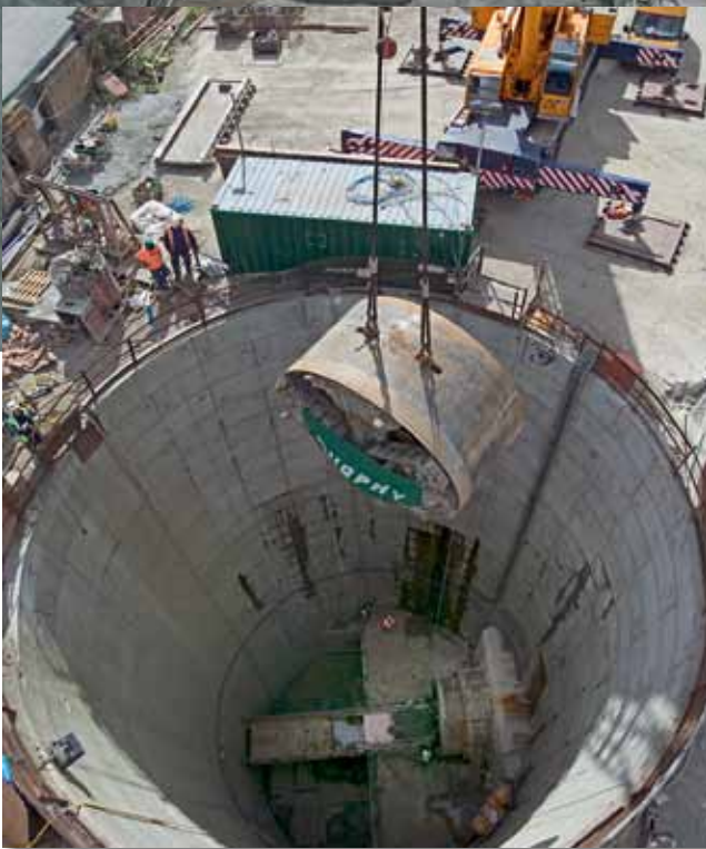
▲ Dismantling and removing the forward shell of "Helen" tunnel boring machine.
